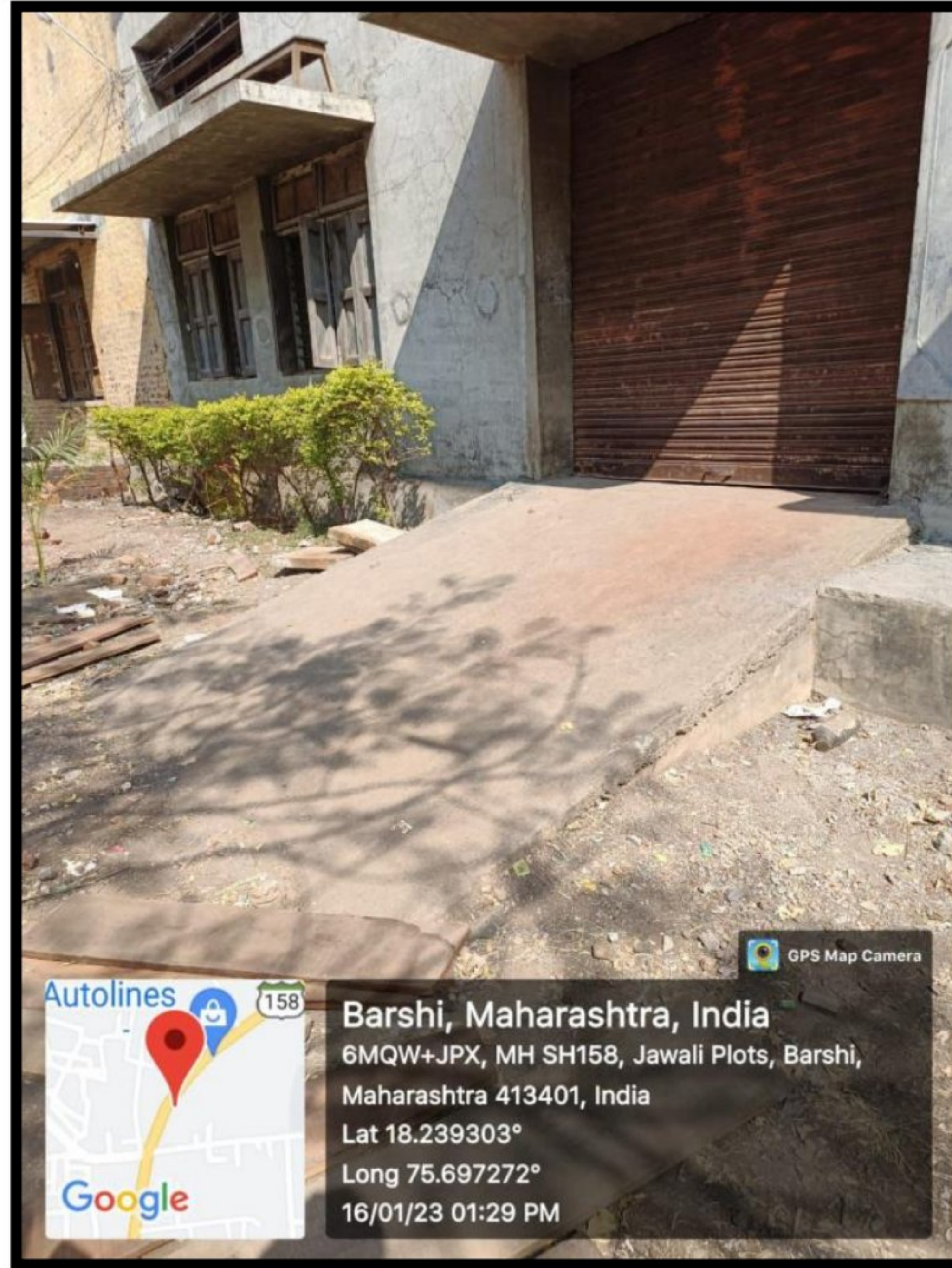
Ramp Facility In Library Building
